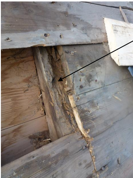
Ingerotte dakspoor i.v.m. lekkage.
