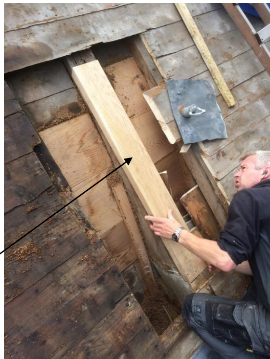
Ingerotte dakspoor i.v.m. lekkage.
